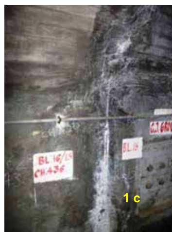
Picture 1 Photograph showing faces of different drainage galleries; a. Dry face in the shear zone in the Lower drainage gallery ; b, c, d. – dry faces of three lower drainage gallery parallel to one another in the construction block joint 15/16
