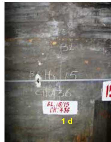
Picture 1 Photograph showing faces of different drainage galleries; a. Dry face in the shear zone in the Lower drainage gallery ; b, c, d. – dry faces of three lower drainage gallery parallel to one another in the construction block joint 15/16
